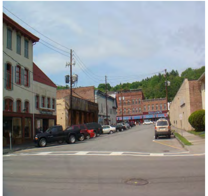
Street with Diagonal and Parallel Parking. In a given space, more parking spaces can be obtained with diagonal parking
