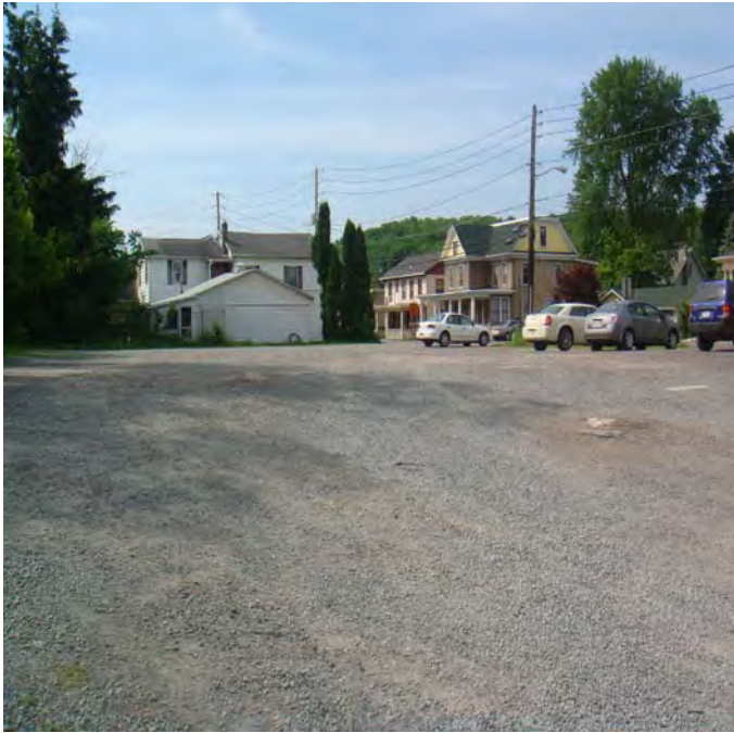
Unmaximized Parking Lot
