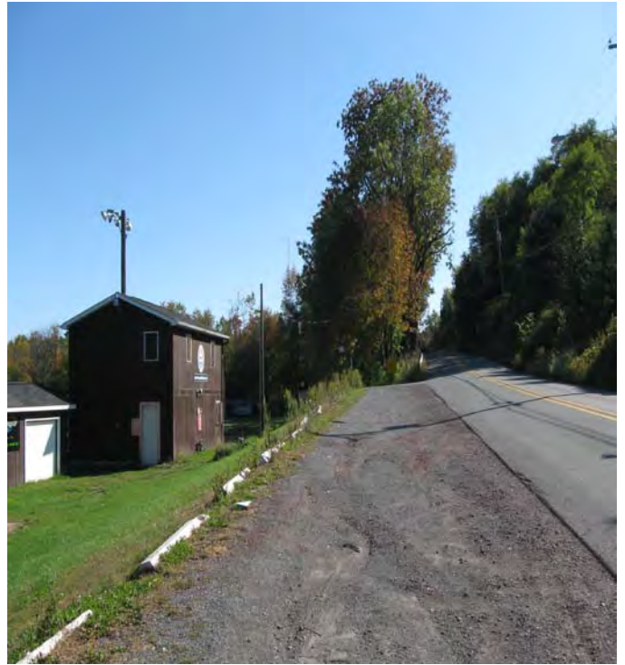
Inadequate Parking at Field
