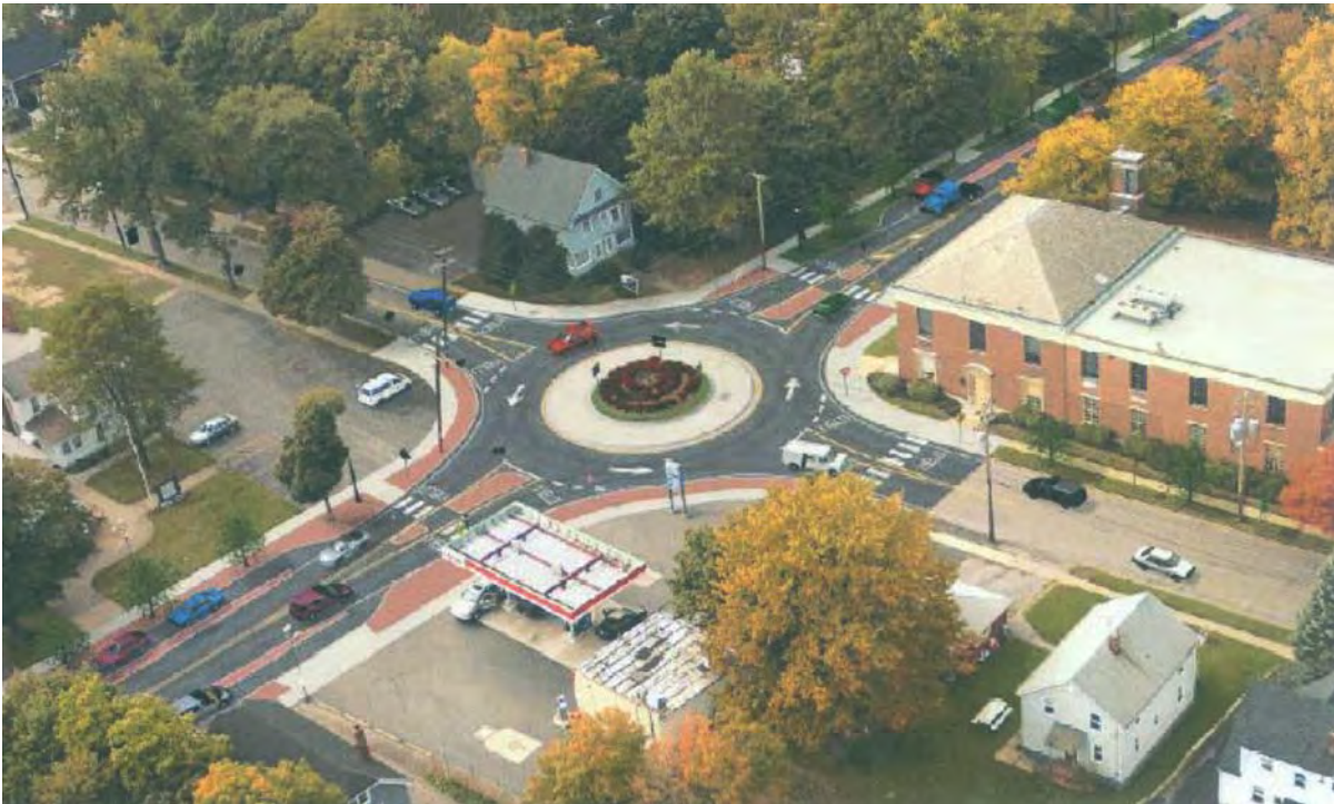
Intersection Before and After Roundabout
