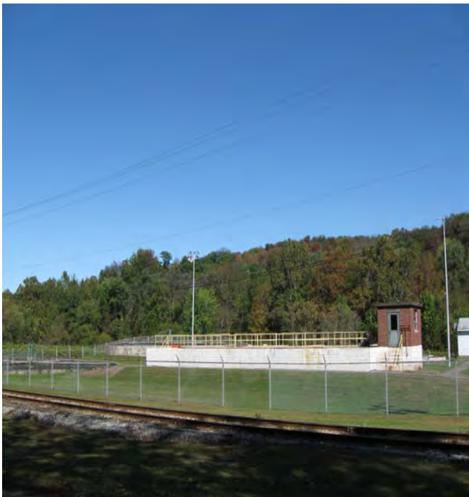
Old Wastewater Treatment Plant - New WWTP Project Underway
